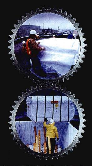
Our patented Lift Liner<sup>™</sup> packaging may be the optimum answer to economic savings for some of your production operations and by-product waste operations. Photos show sludge and sediment removal operation that included; loading of materials into our versatile Lift Liner<sup>™</sup> package, treatment, stabilization, hoisting into our private fleet of railcars and transport to final disposition.
